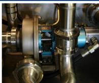
The milk pump, pumps the milk from the outlet of the air separator to the MID meter and the outlet(s) of the installation. This pump can be powered hydraulically or electronically. The pump is placed directly after the air separator.
